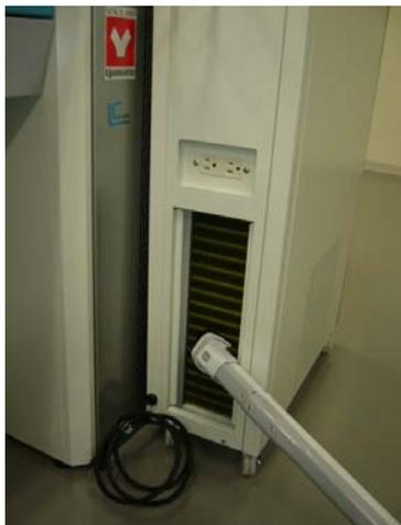
Remove dusts in the condenser fins with an electric cleaner.
